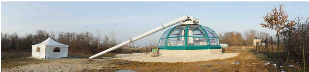
Photo #3: Onshore 3 MW KiteGen® Stem generator in construction by Sommariva Perno (ITA – Dec 2010)
